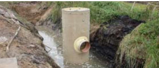
New sluice under construction
